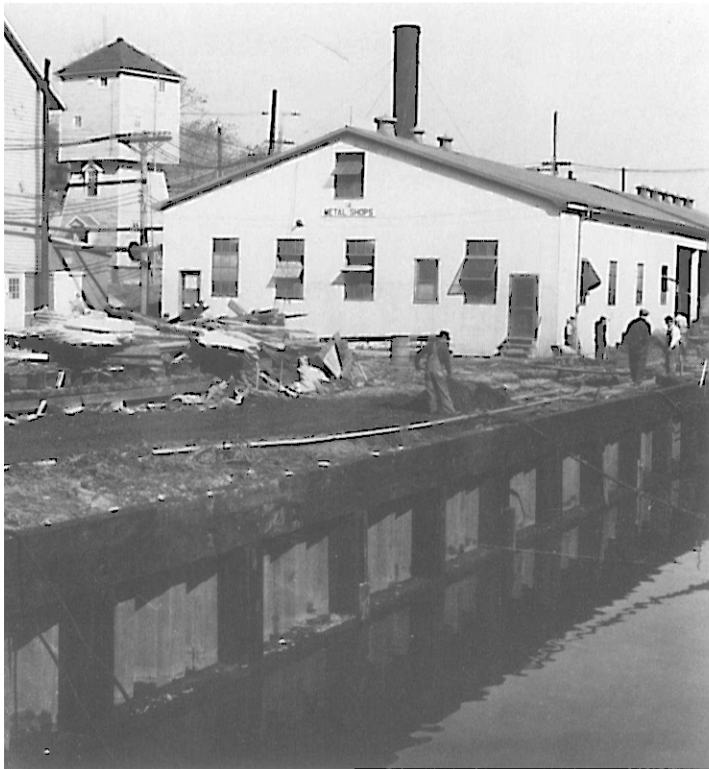
Construction of the shipyard's facilities stepped up in the 1920's and 30's. Bulkhead construction is pictured in the left photo.
