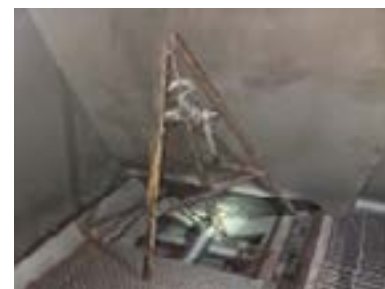
End of the auger supported
