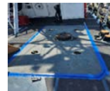
Modified Soft Patch for AC Duct
